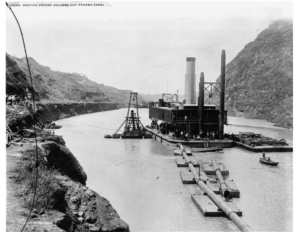
Workers construct Panama canal (around 1910)
